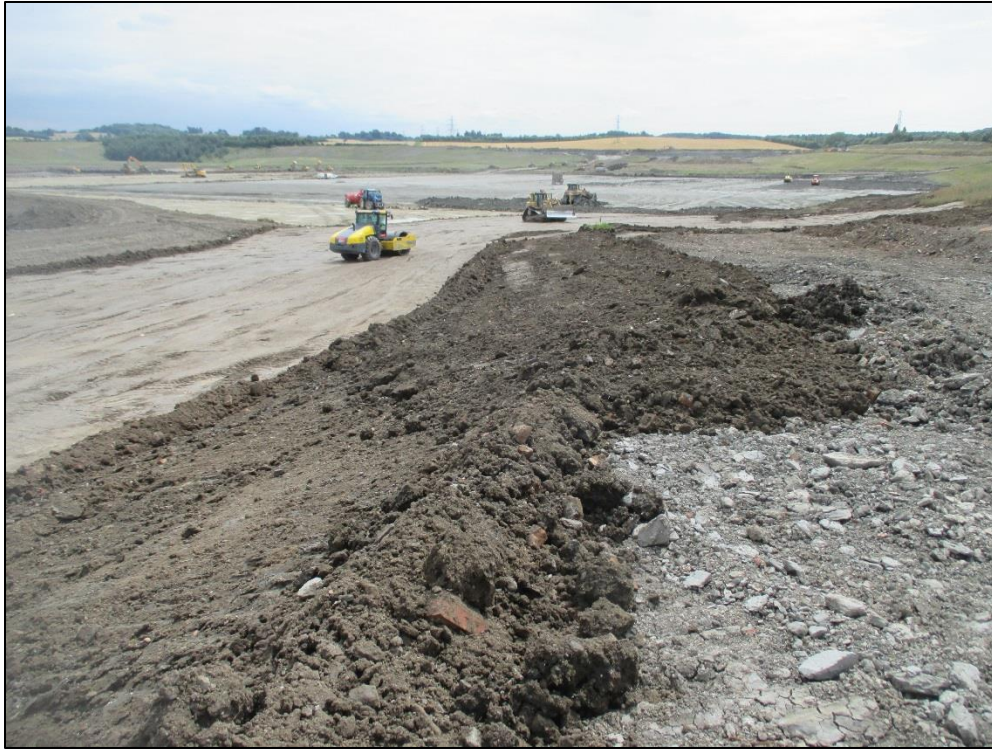
Photograph 1 – Facing broadly south-east across the base of Rookery South Pit.
