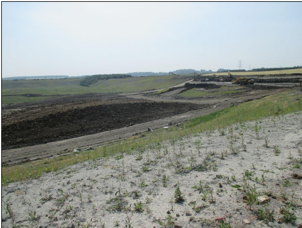
Photograph 4 – Facing broadly south-east from the Electricity Generation Area.
